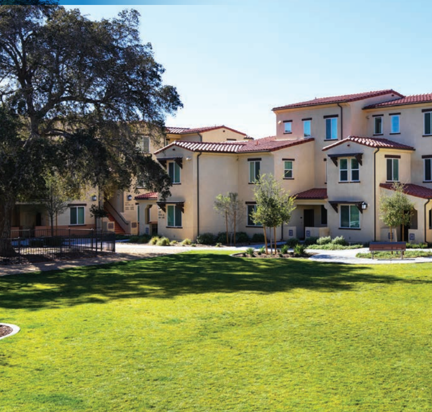
CRESTVIEW TERRACE San Bernardino, CA
